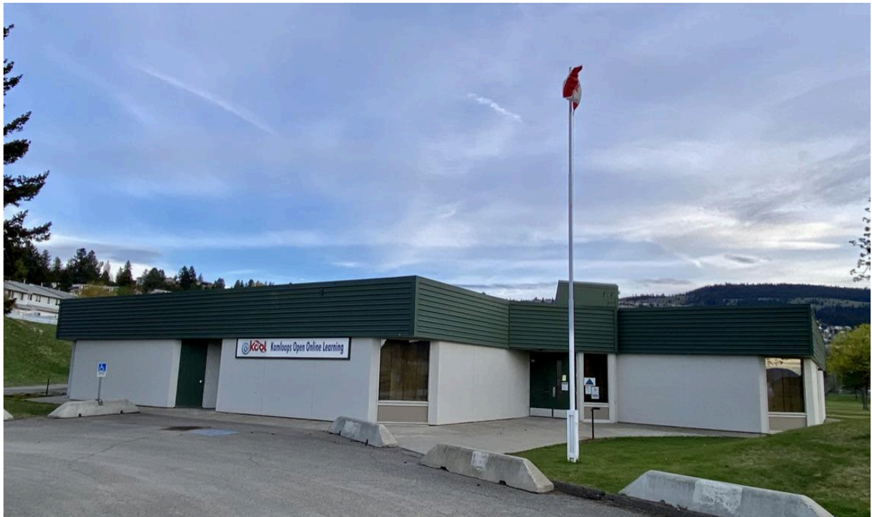
The @KOOL office and secondary program are located within Pineridge Education Centre, pictured above.
